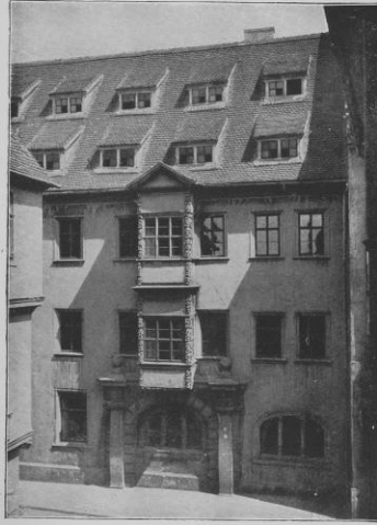
HOUSE OF J. V. WAGNER IN HALLE.
